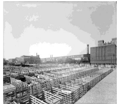
Canada Packers stock yards, south-west corner of Keele Street and St.Clair Avenue West.
